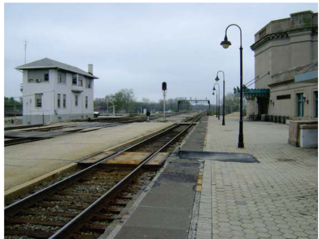
Looking south from the BNSF N TRK (UD Control Tower left, Union Station right)
